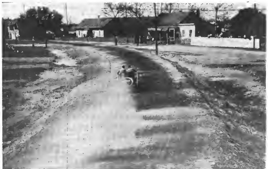
One of the Banked Turns Especially Prepared by the County Road Commissioners.
